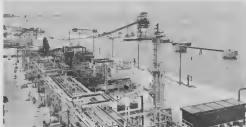
View of Lago's HDS Pier, used for sulfur loading and for unloading heavy equipment for the new HDS units.
